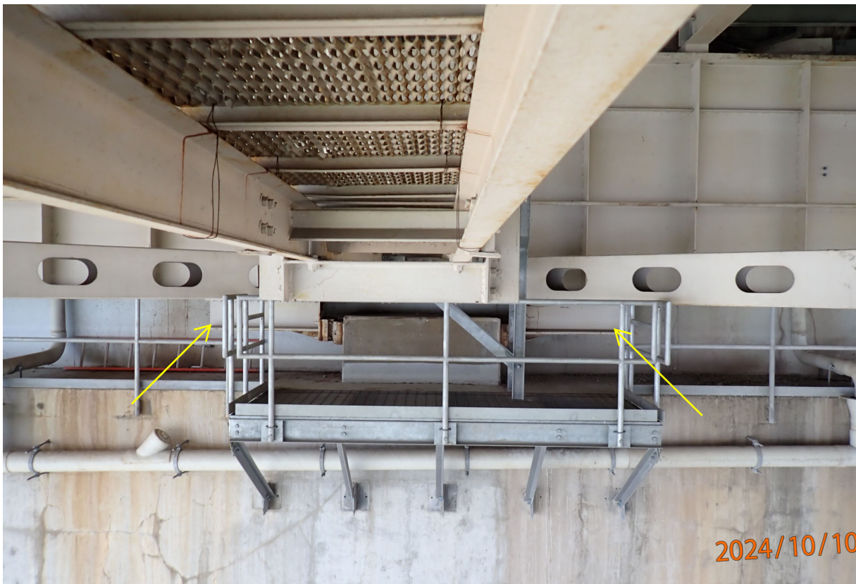
Closer view of previous photo
