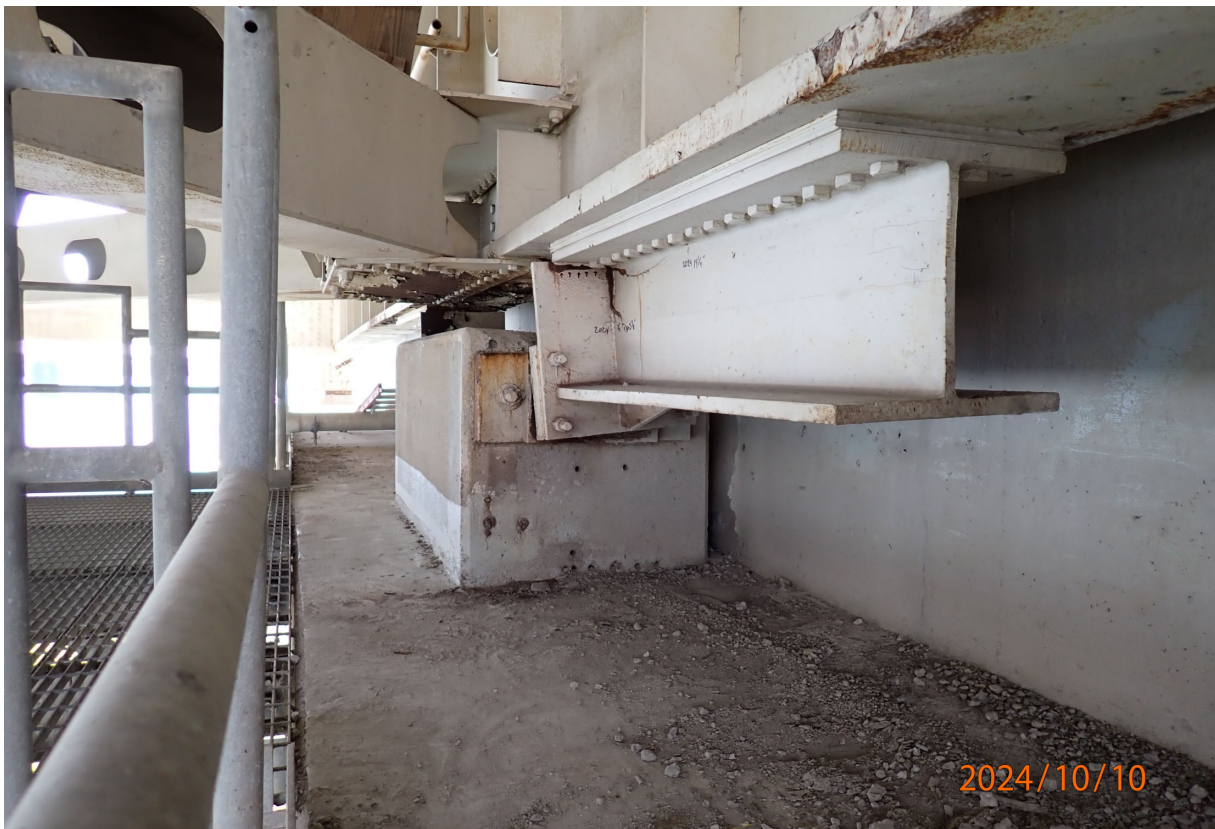
East wind shear beam at Floorbeam 0', Pier 6 (south face, looking west)
