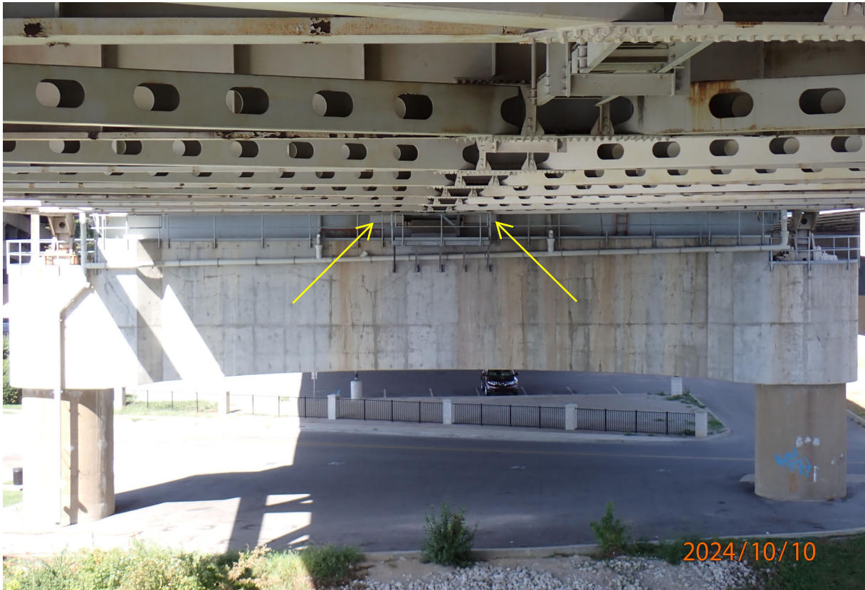
South face of Pier 6 showing location of wind shear beams
